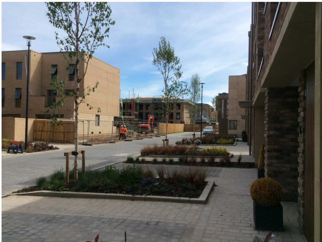
Robert Street looking south. May 2017. Work is in progress on Bayldon Square.
