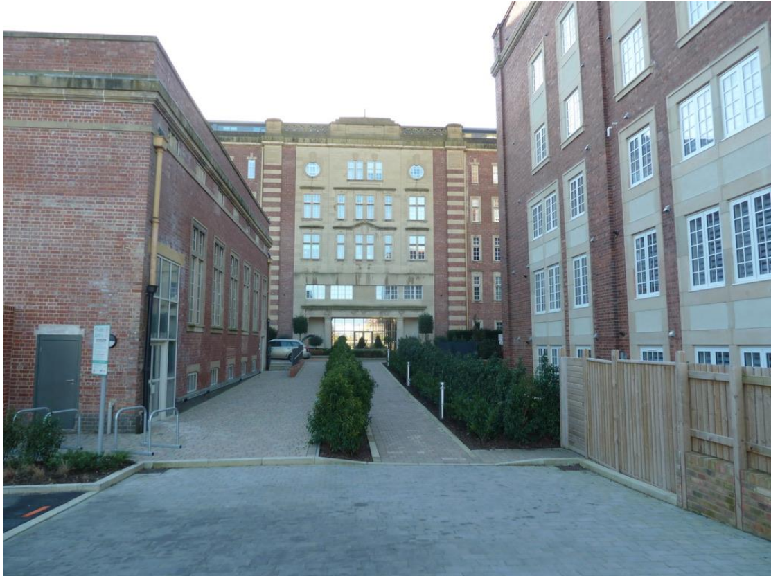
Footpath between the Liquor Store (left) and the Boiler House (right), January 2023.
