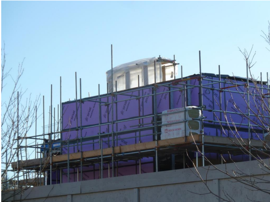
Construction in progress on the Brainkind building, 2023.
