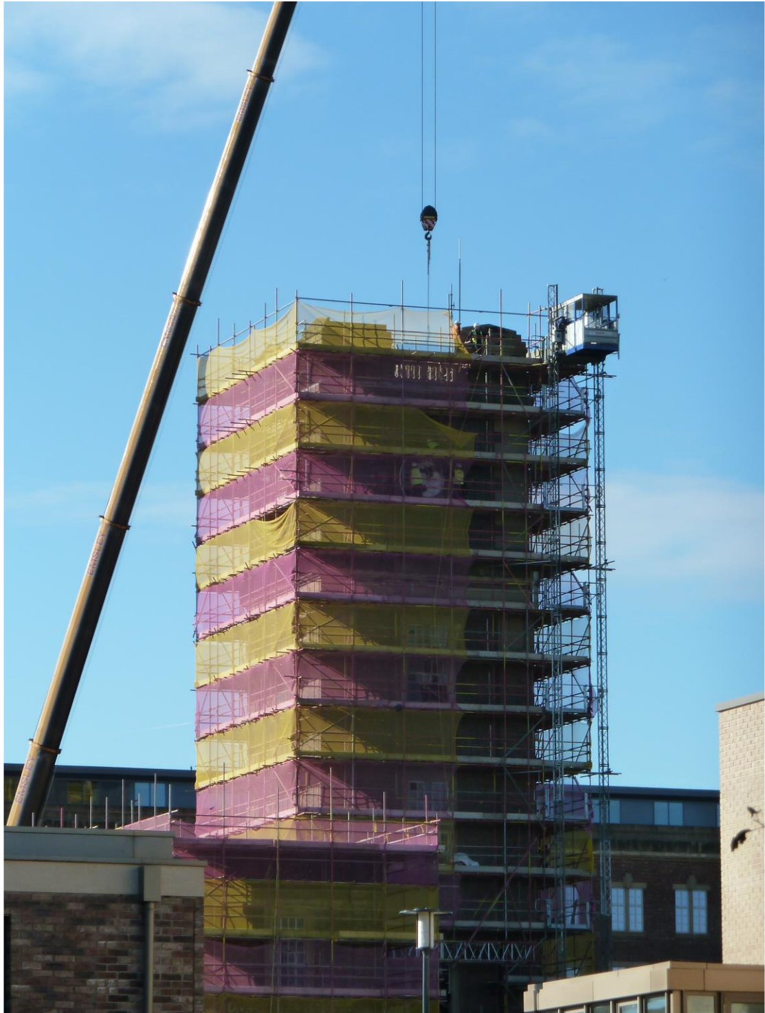
Work on the Clock Tower in 2018.
