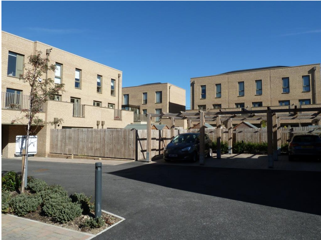
Parking courtyard off Clock Tower Way, September 2018.
