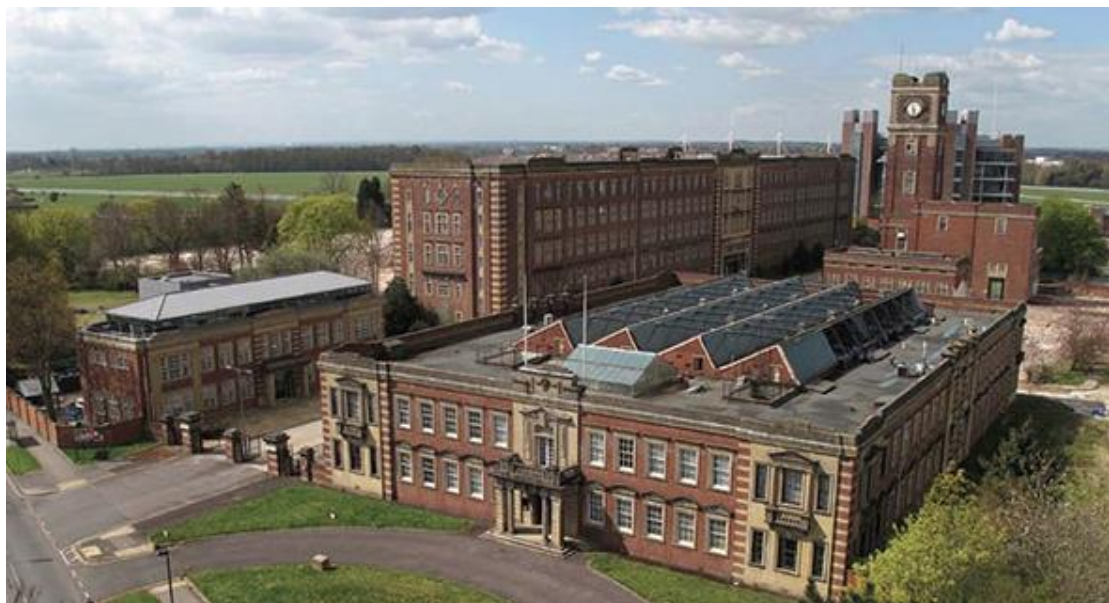
This photograph shows what the southern end of the site looked like once the clearance process had been completed. Source: Planning documentation, 2012.
