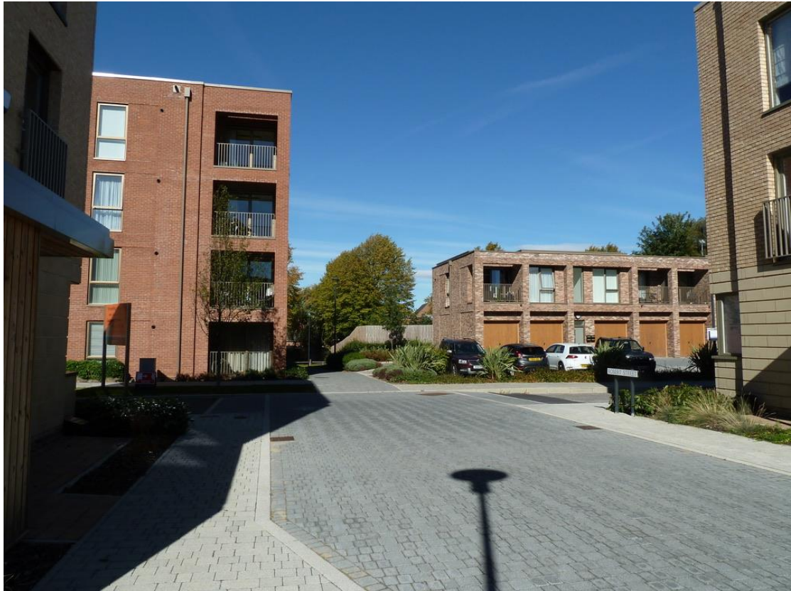
Neapolitan House (left) and Bayldon Court (right), with ramp down to Campleshon Road. Taken from Robert Street, 2023. The former comprises 18 apartments; the latter is a group of four one-bedroomed apartments over garages.
