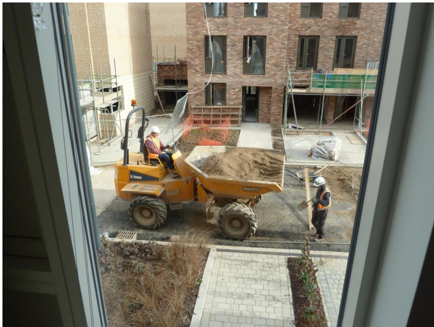
Robert Street. Block paving in progress in November 2016.
