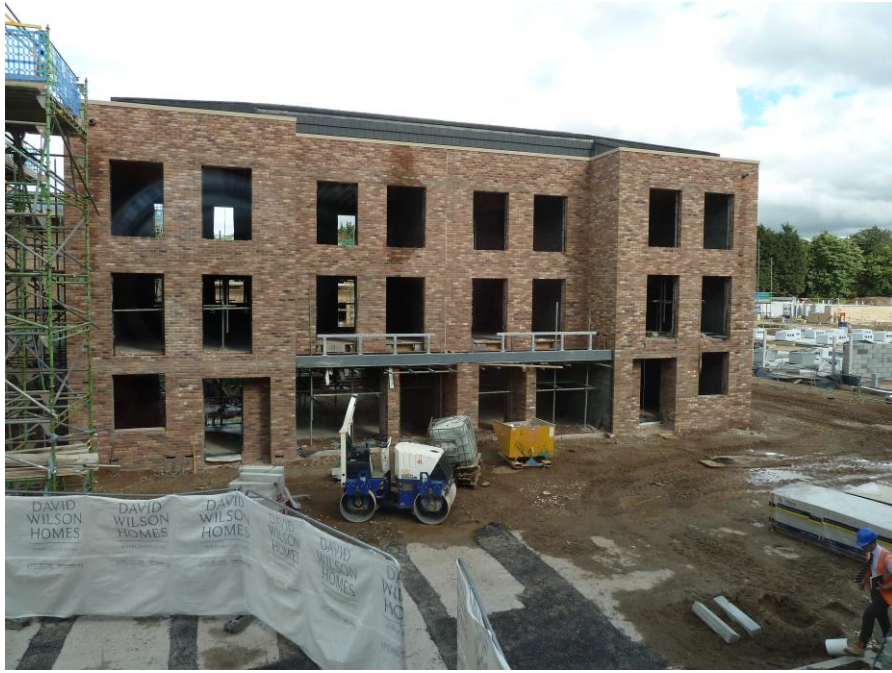
East side of Robert Street under construction. August 2016.
