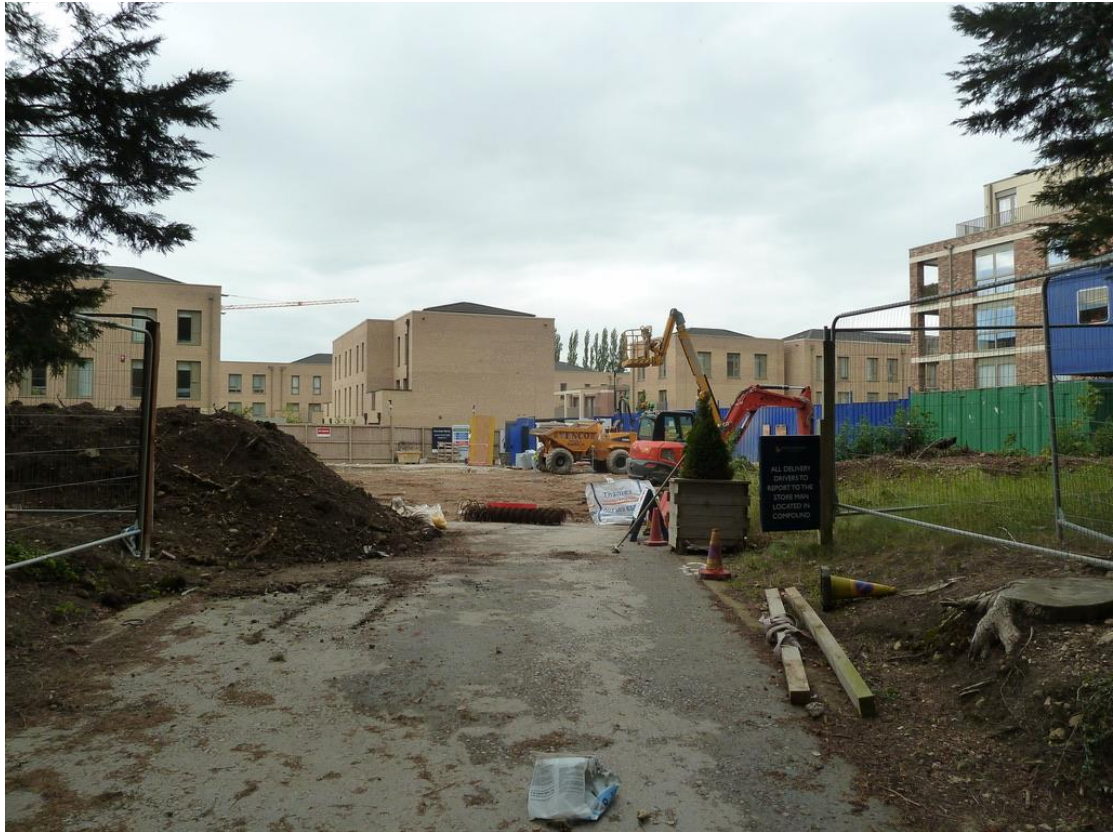
Preliminary works on Thistle House as viewed from Bishopthorpe Road, August 2020.
