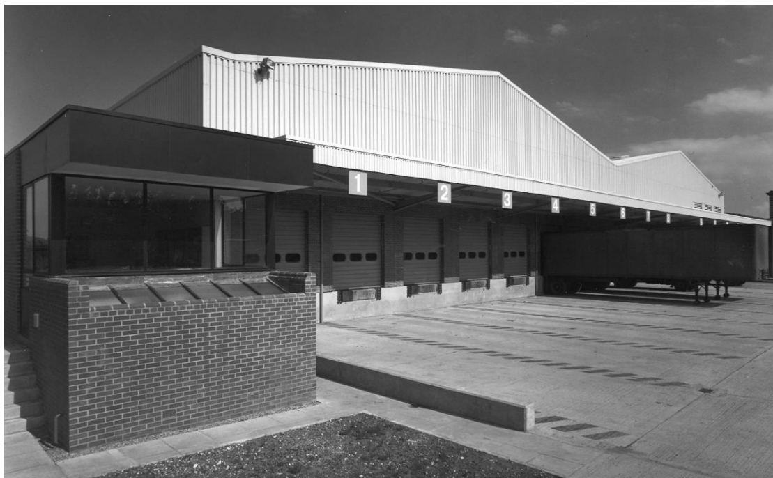
This photo shows the newly completed distribution depot and the northern end of the site. From here, large trucks would arrive and depart carrying Terry's products throughout the UK and beyond. Taken in 1975, courtesy of York Press.
