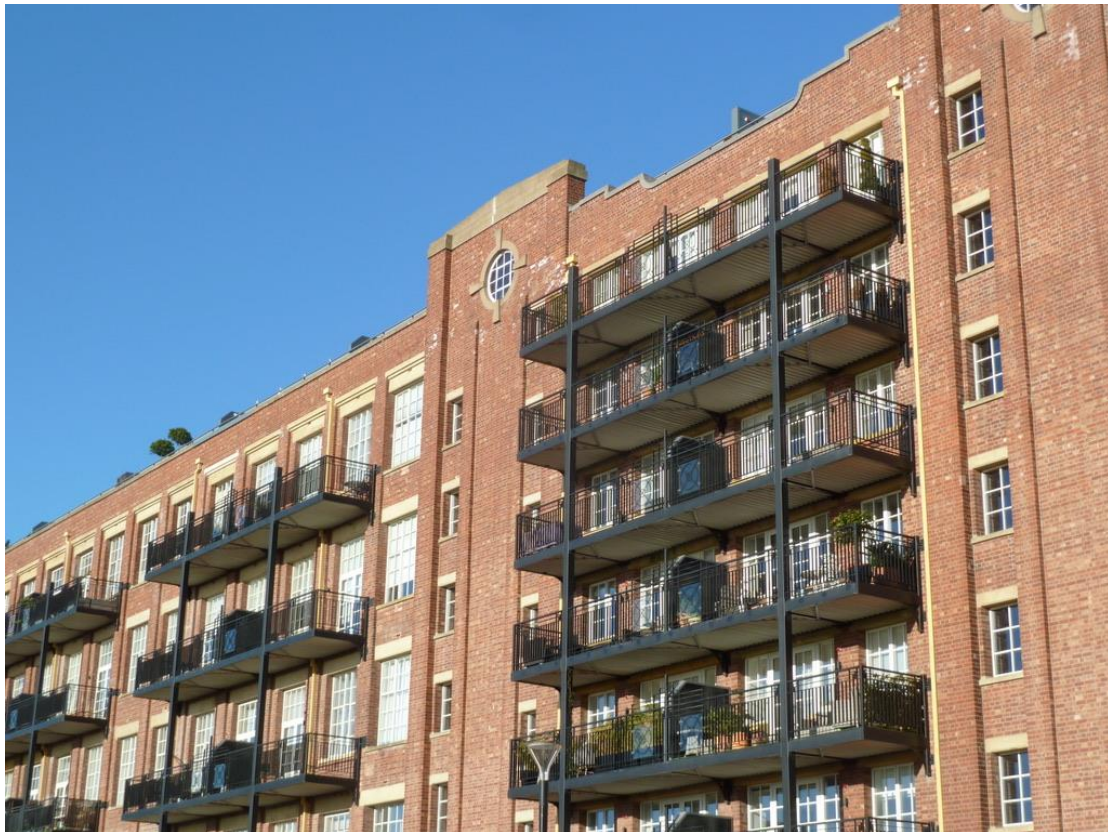
South-facing aspect of The Residence (January 2023).
