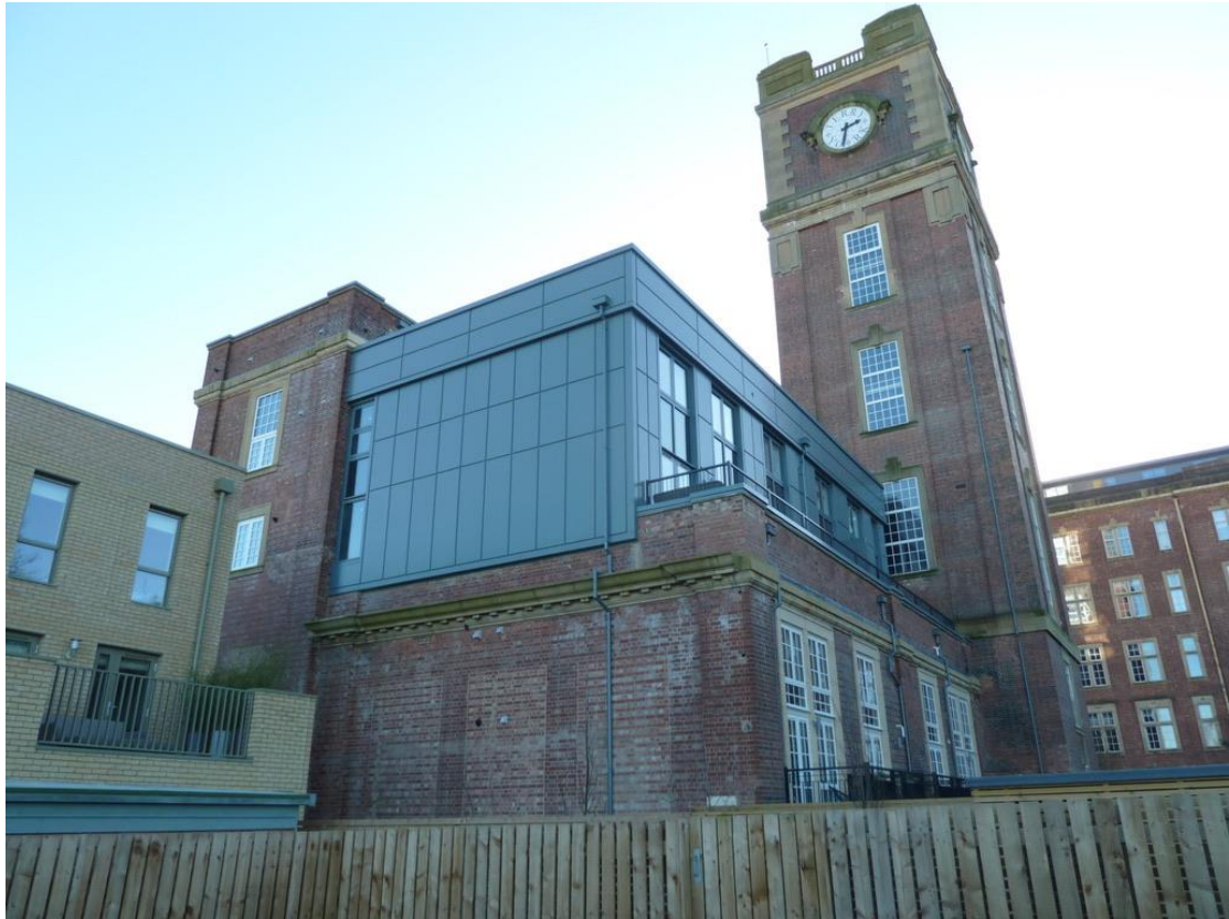
The Boiler House apartments, January 2023.
