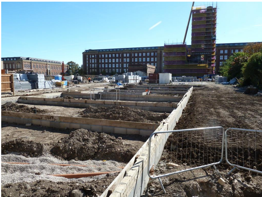
The southern extension of Clock Tower Way under construction, September 2018.
