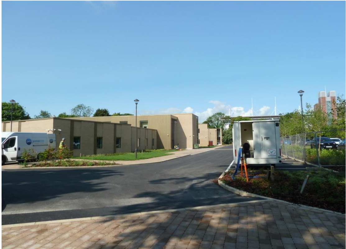
Brainkind nearing completion, 2023.
