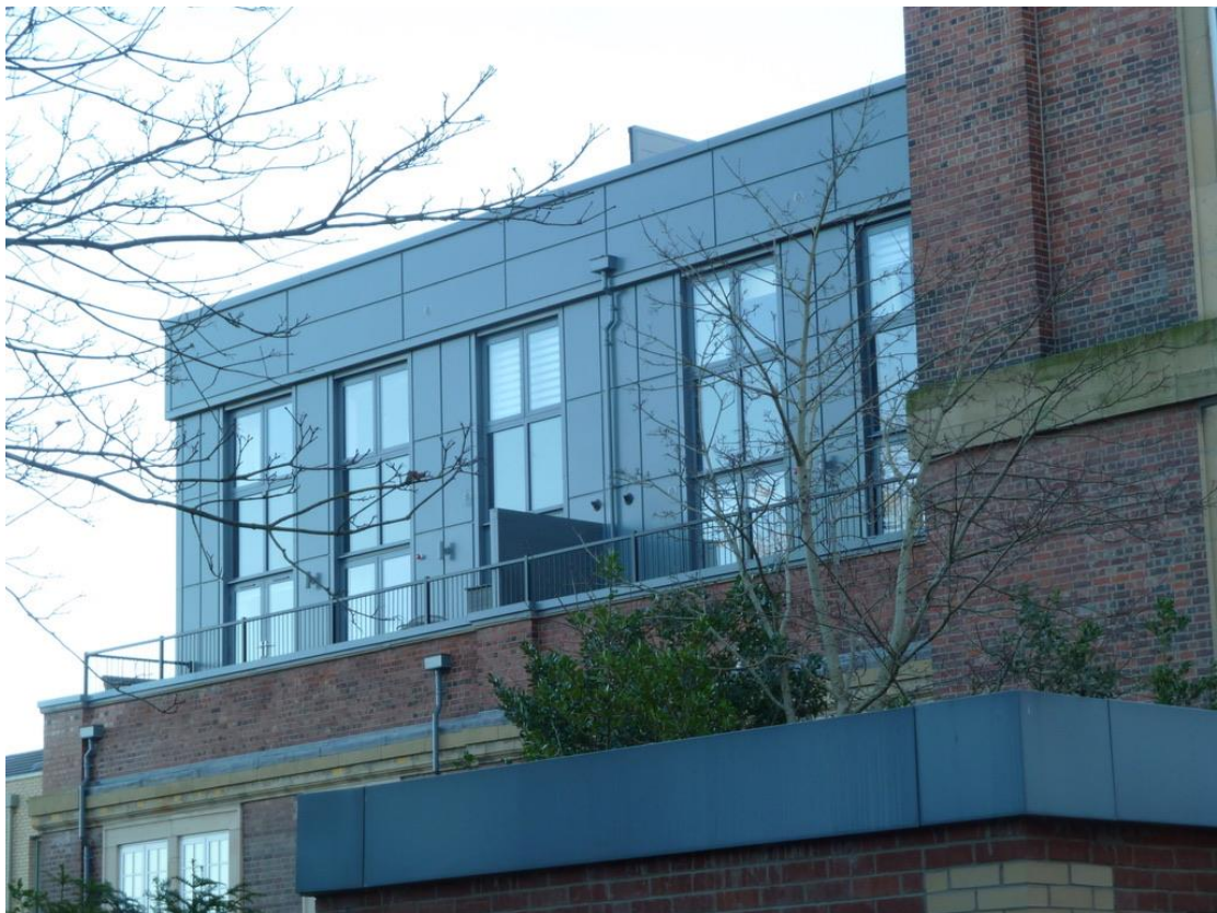
Clock Tower and Boiler House, January 2023.
