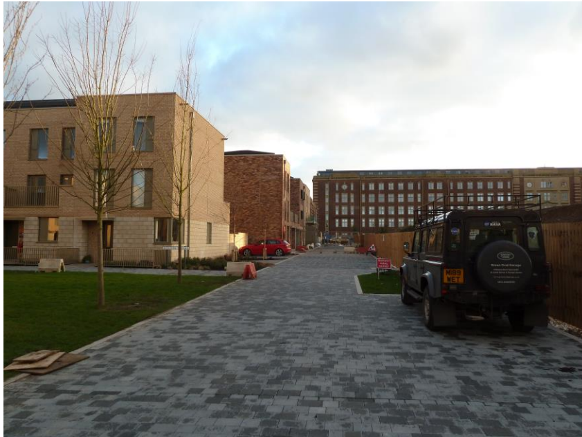
February 2018. View south from Bayldon Square (on the left) towards the main Terry's Factory.
