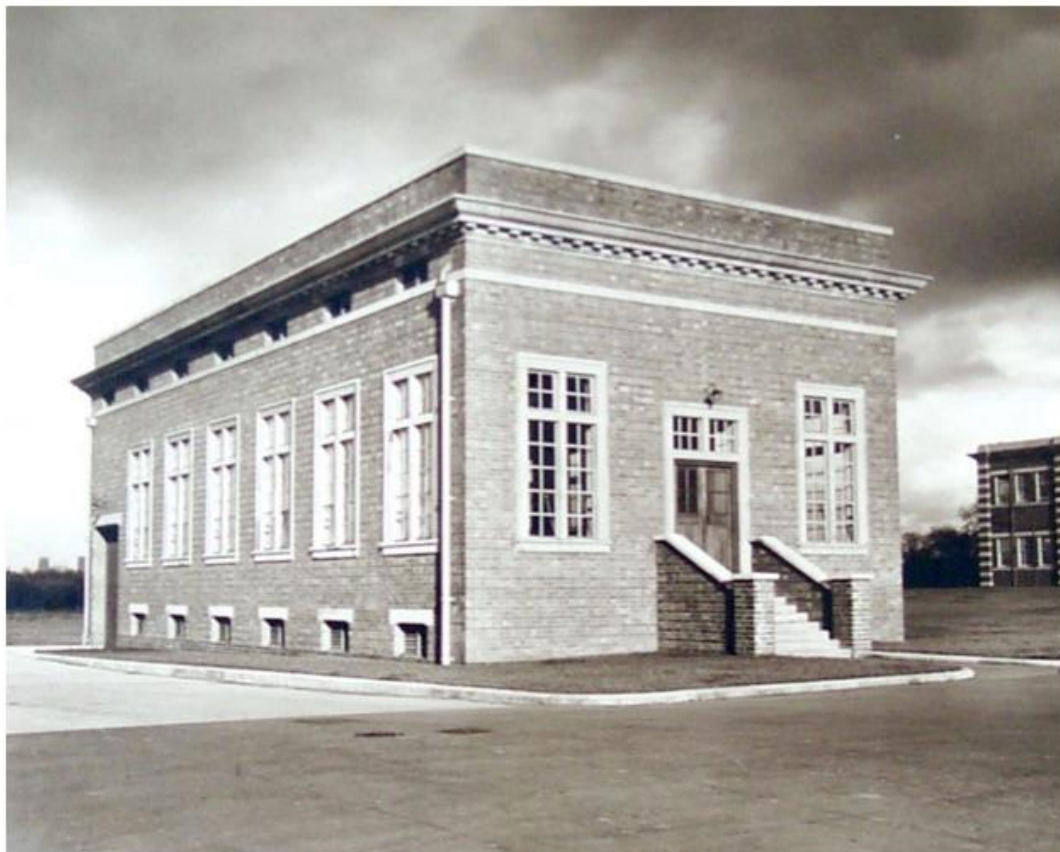
All powered up: the electrical transformer house
