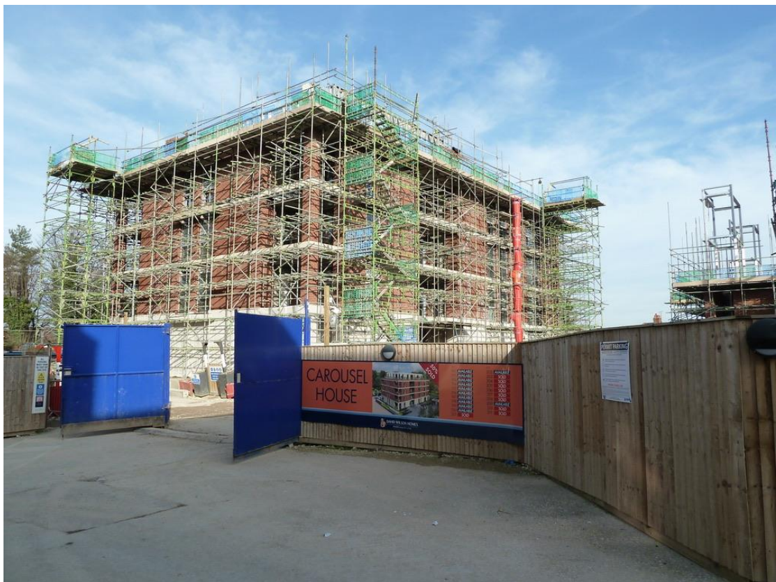
Carousel House with main structure complete, February 2019.
